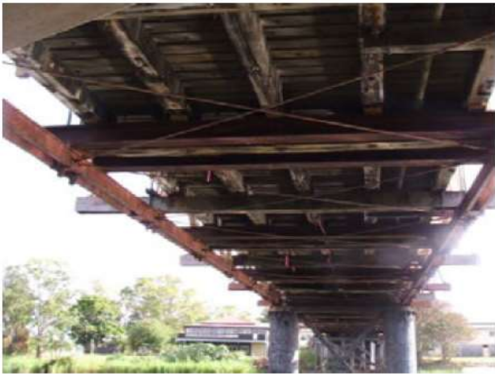
Plate 4.1 View north showing underside of Sportsmans Creek Bridge
