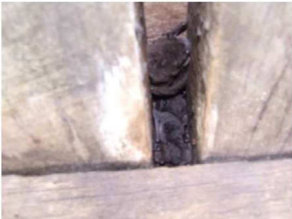
Plate 4.3 Large-footed Myotis in bridge decking
