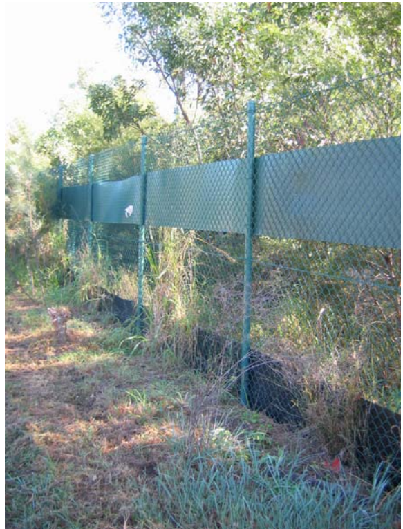
Fencing which is designed to prevent animals from climbing over the fence or burrowing beneath it to enter the roadway.
