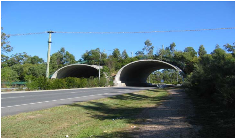
One of Brisbane's vegetated land bridges linking two areas of bushland otherwise separated by a road. A rope bridge for arboreal mammals is located beside the land bridge.
