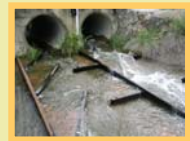
Prototype #3 Solander Road pipe culvert fishway
