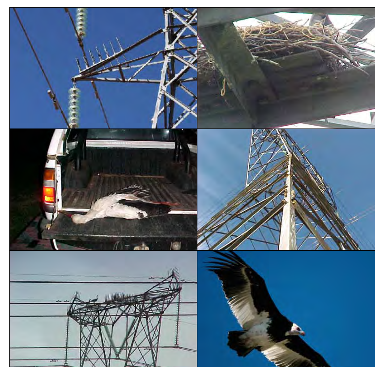
Image 2 top left: Final bird guard design
