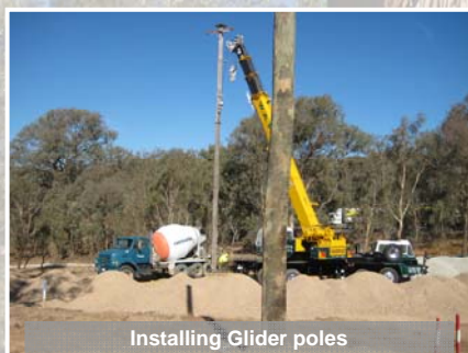
Installing Glider poles
