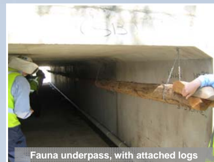
Fauna underpass, with attached logs
