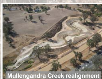
Mullengandra Creek realignment
