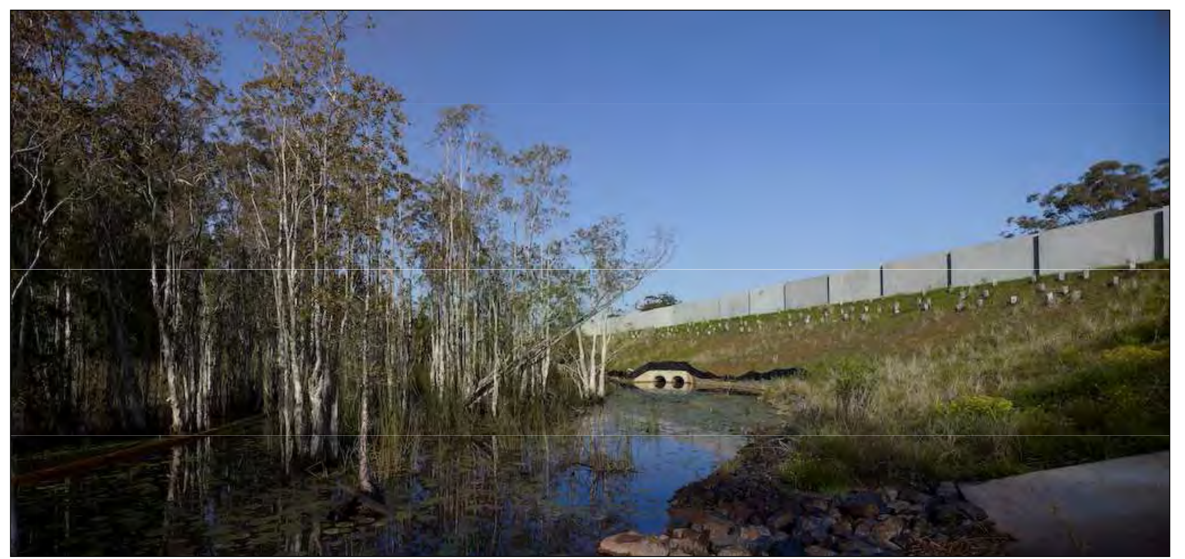
Figure 2: Hydrological Connection Measures including rock mattresses through the embankment and culverts for high flows and aquatic fauna: Bonville Bypass NSW.
