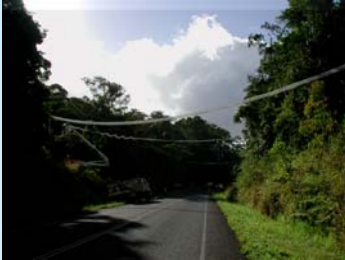
Palmerston Highway Canopy Bridges
