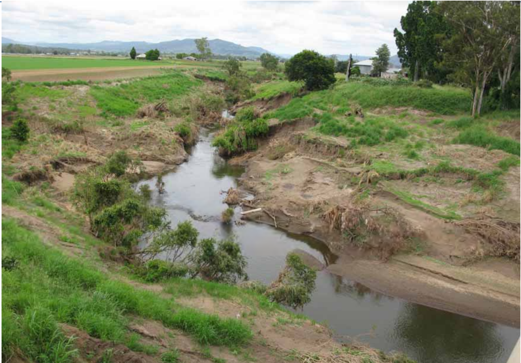
Tenthill Ck upstream of Gatton-Helidon Road Bridge
