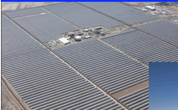
Andasol 1, Spain, 50 MW, 7.5 hr storage
